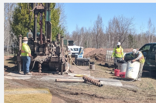
> Geotechnical work being performed along Line 5 Wisconsin Segment Relocation Proposed Route.
